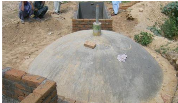
Figure 52 Fixed Dome Type
